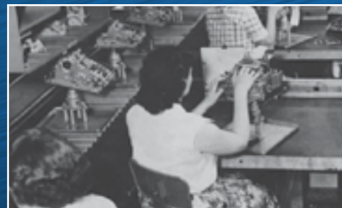
POW-R-ARMS have been popular in production lines for decades. Seen here in use at Burroughs Corporation, circa 1956.
